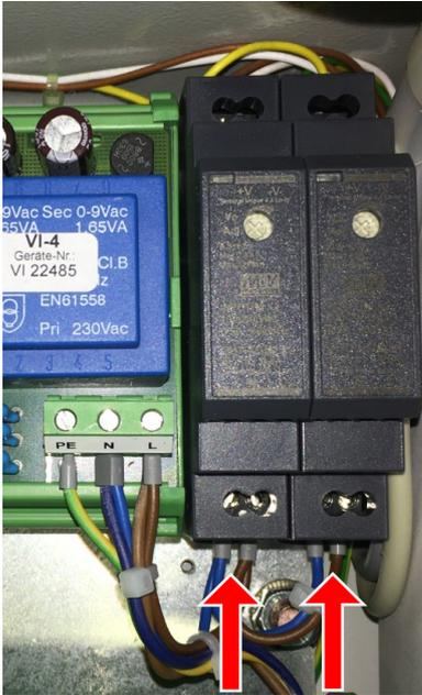
Figure 20: Power supply units, fixing
