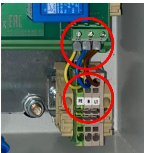
Figure 19: Power supply terminal
