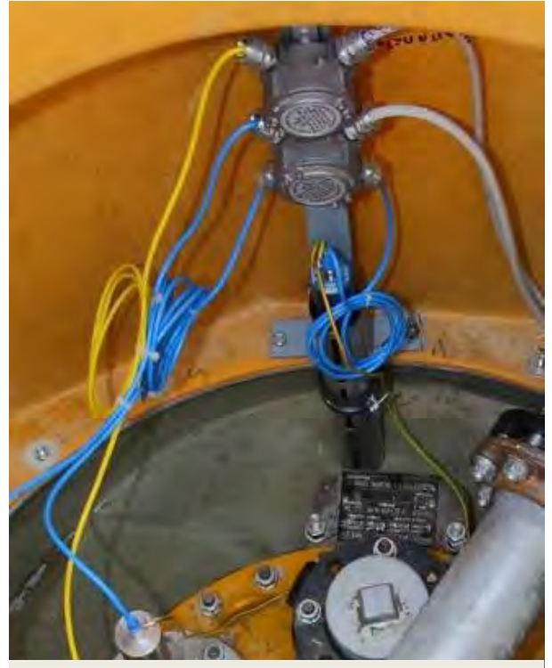
Probe wiring complete !
