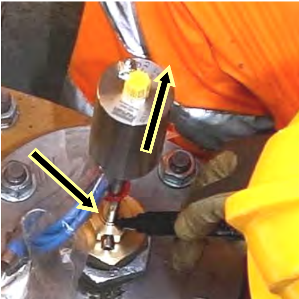
Mark the "Bottom Position" and pull out the probe
