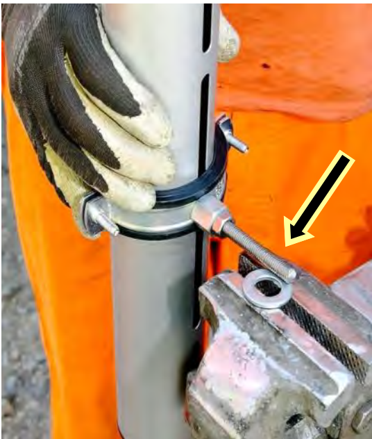
Mounting example with washer welding by installer
